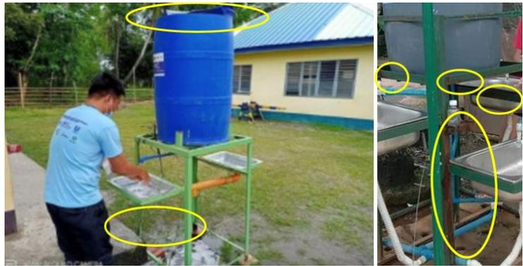
Photo from left to right: a handwashing facility with damaged plastic drum with no cover and no pipe connection from the sink to drain wastewater; handwashing facility with rusted soap handler and steel holding the plastic drum and sink.
