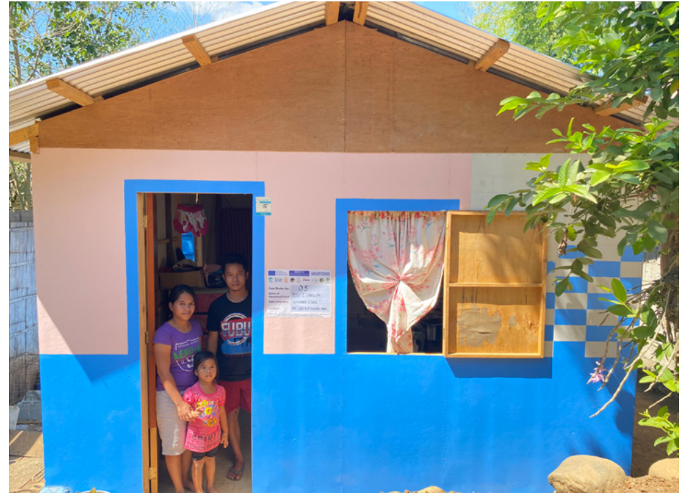
Dianne and Jojo, together with their daughter, pose inside their newly built core shelter as part of the REACH 3 Project's Abra Earthquake Response. Their house was totally damaged when a 7.0-magnitude earthquake hit their province.
